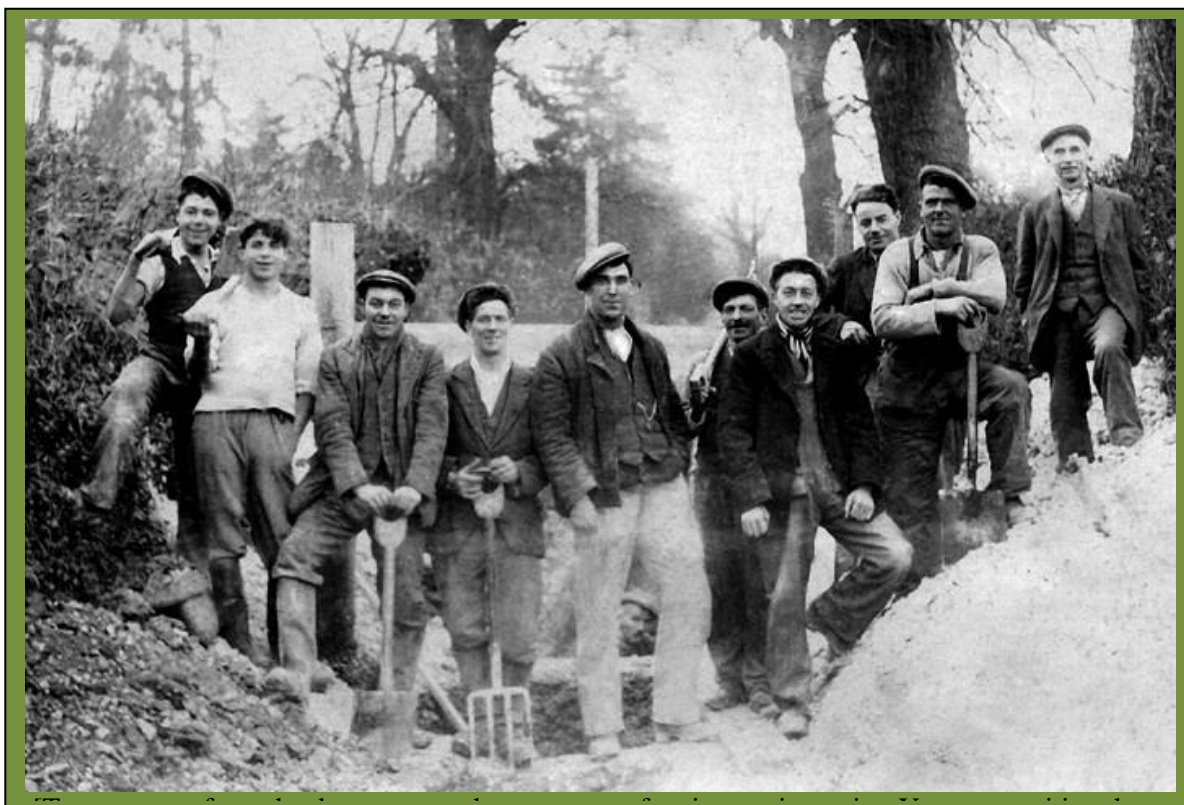
Digging the main sewer.
